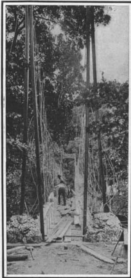
The Bridge as Viewed from the North Bank. Note the Steel Rail Towers.
