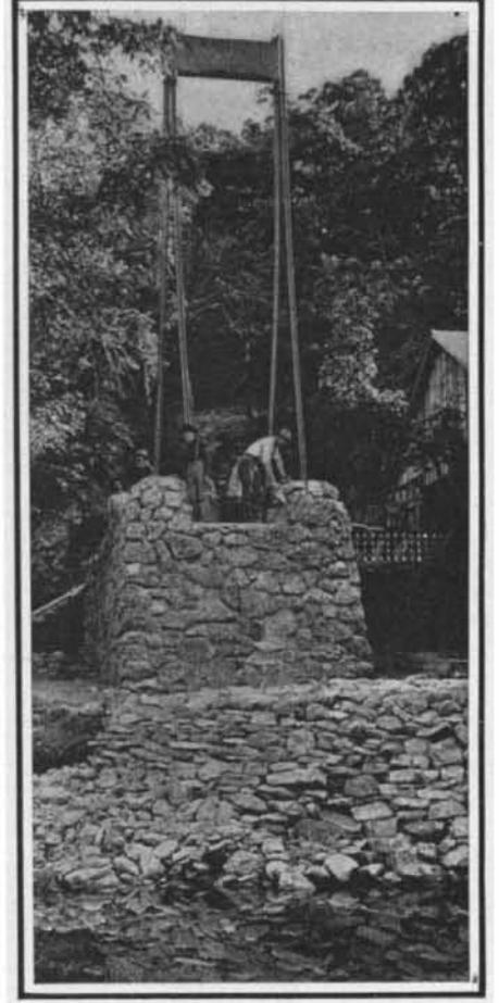
The Towers Consist of Four 70-Pound Railroad Rails Set in a Concrete Base.
