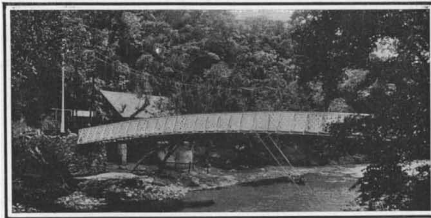
The Completed Suspension Foot Bridge across Rock Creek, Platt National Park.
