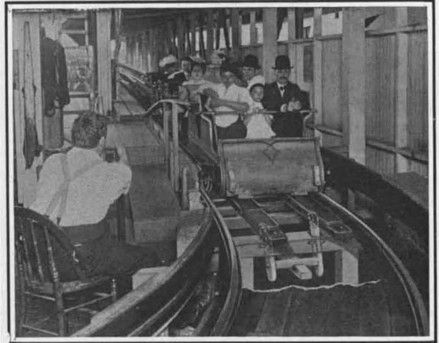
Lifting Car Off the Rails Onto Friction Beams.
