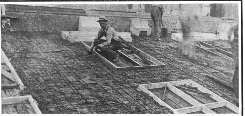
Laying the reinforcement of the walls.
