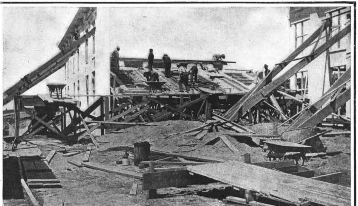
Two walls in position. Intersecting wall under construction.
