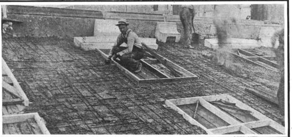
Laying the reinforcement of the walls.
