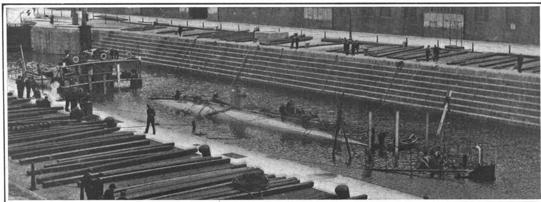
FLOATING A SUBMARINE INTO A VESSEL FOR TRANSPORTATION.
