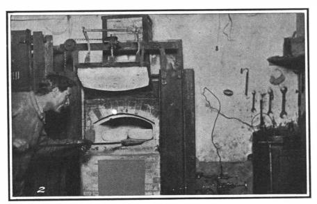
Thrusting the crucible into the furnace.
