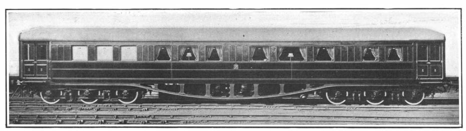
The royal car is 67 feet long, 9 feet wide, and 12 feet 11 inches high from rail level to roof. The strong steel underframe adds to the car's collision-resisting ability.
