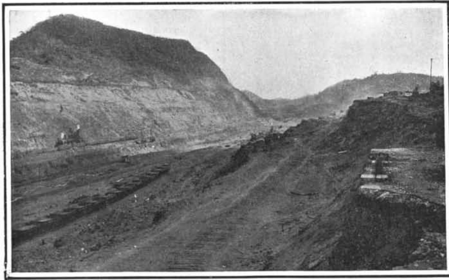
Culebra cut, looking south.
