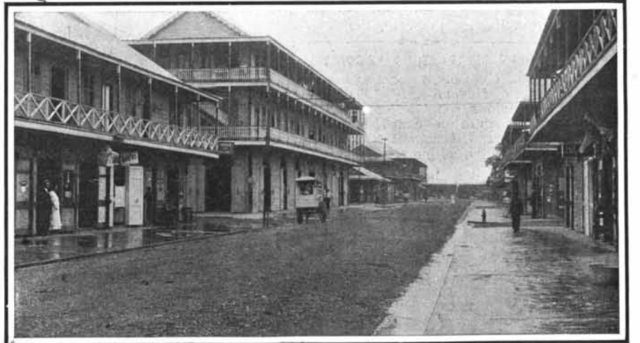
Tenth Street, Colon, after paving.
