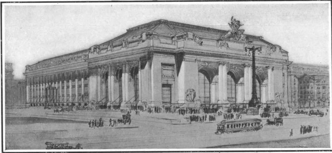
VIEW OF THE NEW GRAND CENTRAL STATION FROM FORTY-SECOND STREET.
