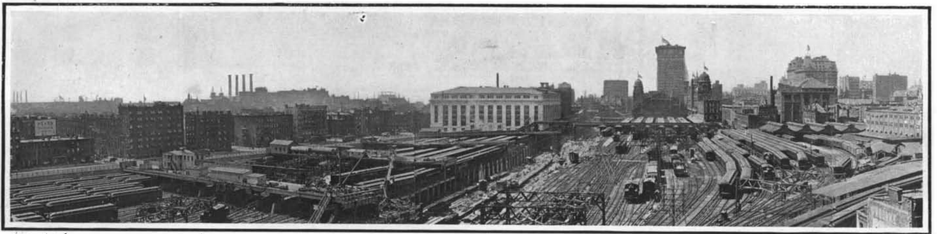
The completed portion of new yard.
