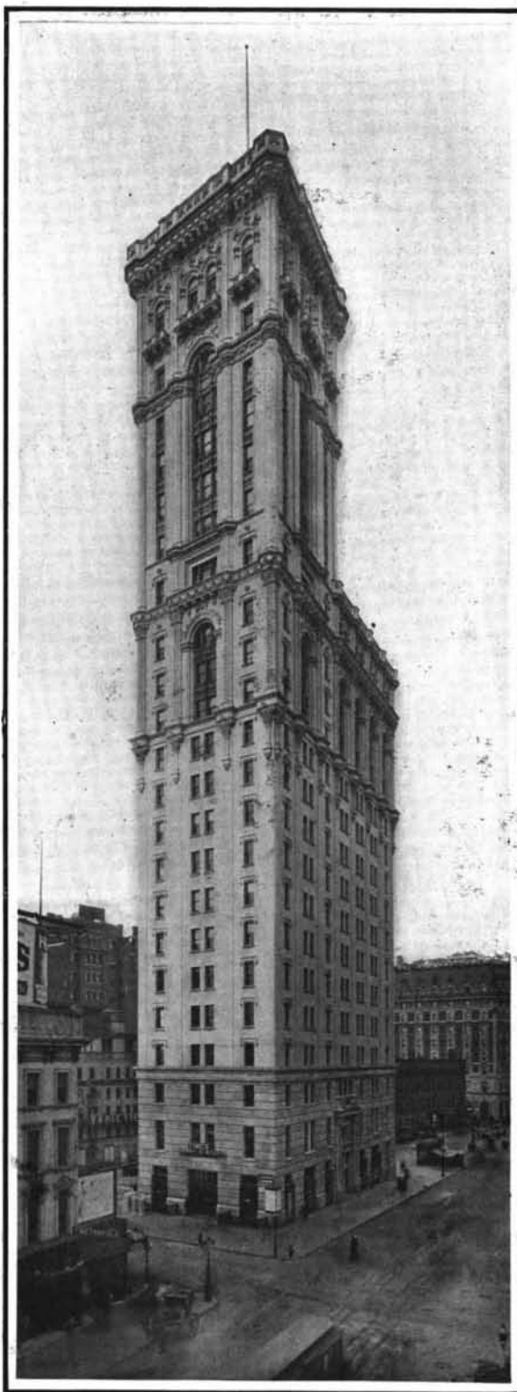
Rises 363 feet above a triangular base. There are 23 stories in the tower. Total floor space, 117,000 square feet. Copyrighted 1906 by Irving Underhill.
