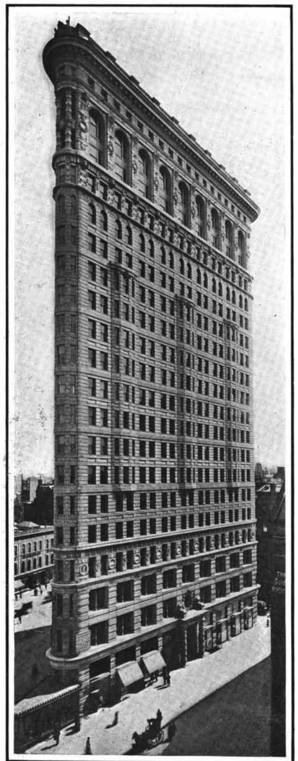
Popularly known as the "Flatiron." This building, 310 feet high, stands on a triangular base measuring 215 feet on Broadway, 198 feet on Fifth Avenue, and 86 feet on 22d Street. The site cost $2,500,000. Copyrighted 1903 by Irving Underhill.
