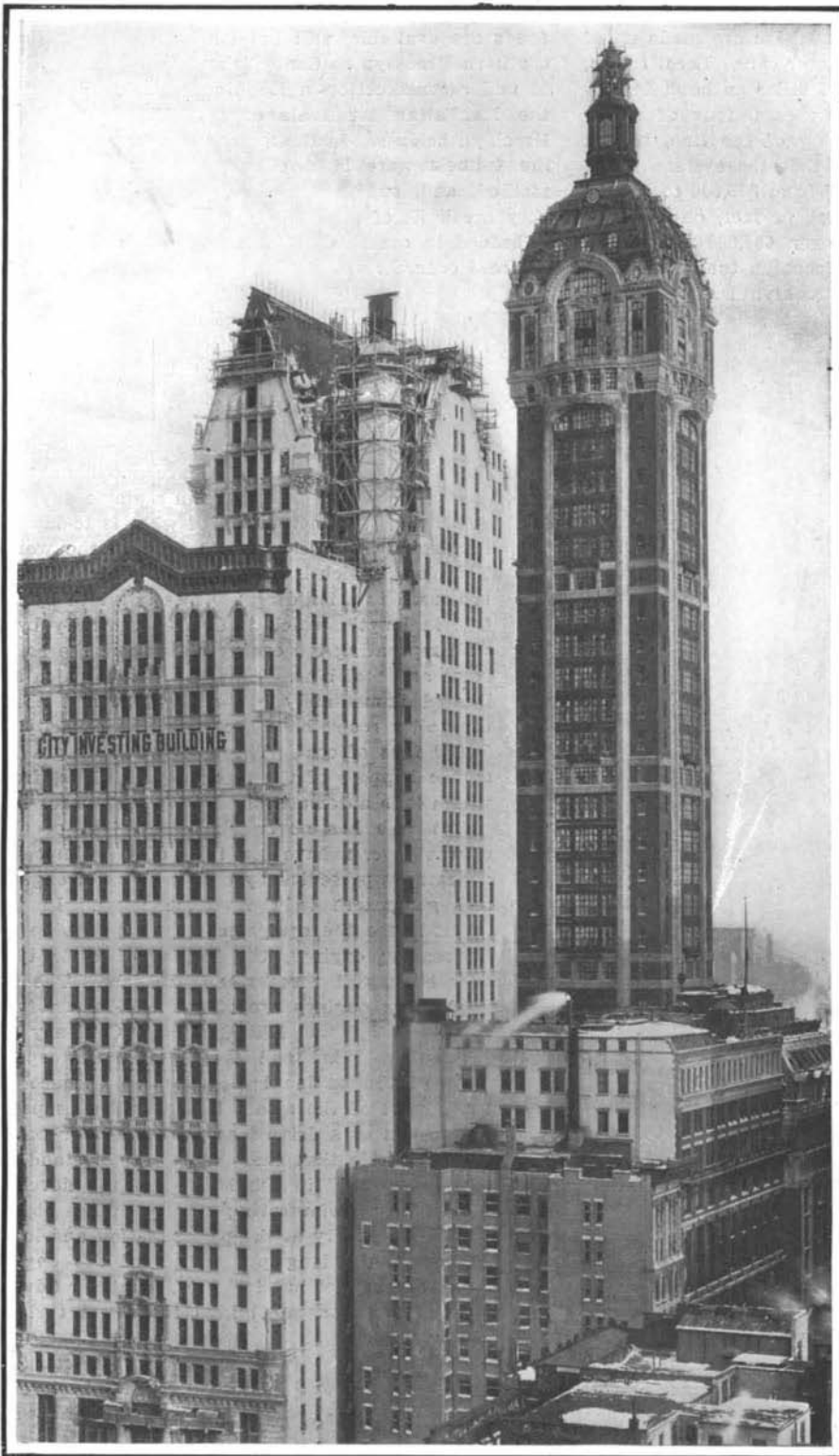
The City Investing Building, 435 feet high, contains 31 rentable stories. It covers a lot 124 feet by 308 feet, and its total floor area is 670,000 feet.
