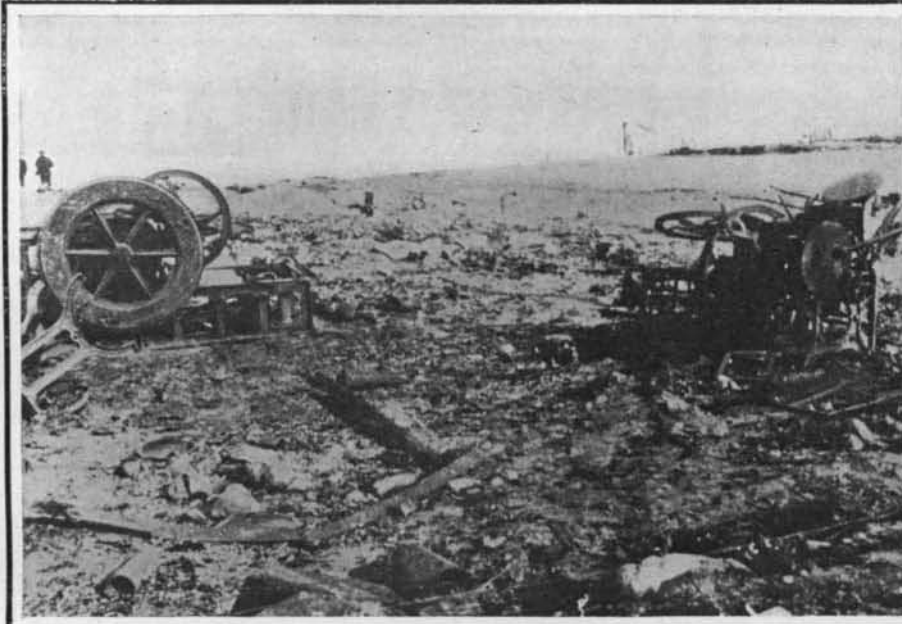
The destruction wrought by forest fire in a western village—only the machinery of a factory left.
