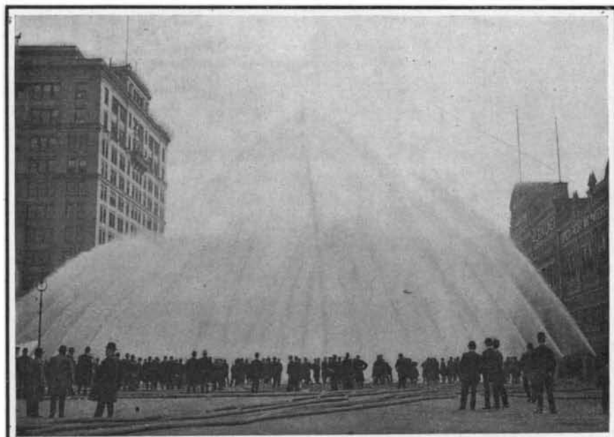
Twenty-six high-pressure streams discharging a volume of water sufficient to extinguish any single fire.
