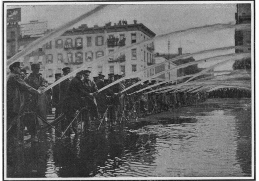
Using the spider-legged nozzle holders in a test of the high-pressure fire service in New York.
