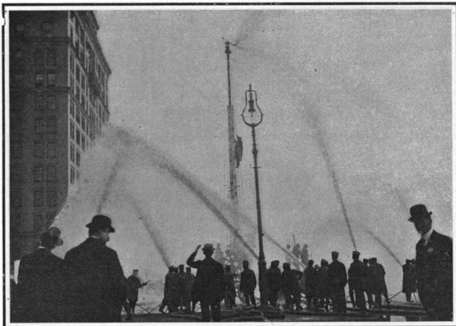
High-pressure streams from water tower and nozzles mounted on holders can be thrown easily above a twelve-story building.
