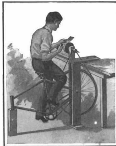
A SIMPLE FOOT-POWER GRINDER.
