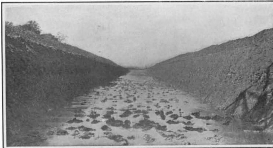
Section of Canal Excavated in Soft Material. The Material Dredged Out and the Earth Excavation Amount to on the Whole Canal 112,665,700 Yards.
