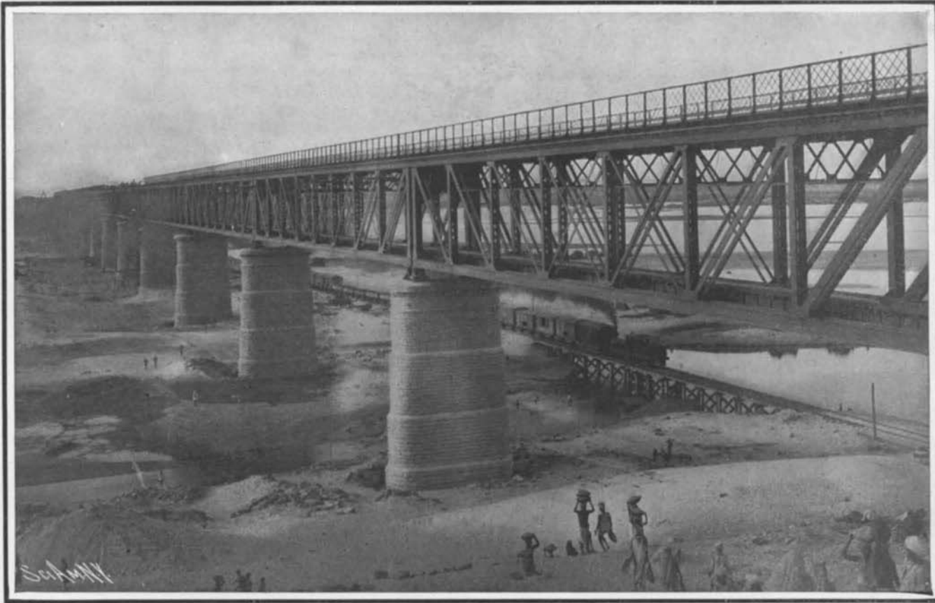
The Curzon Bridge Practically Completed, Showing Temporary Line in River Bed.
