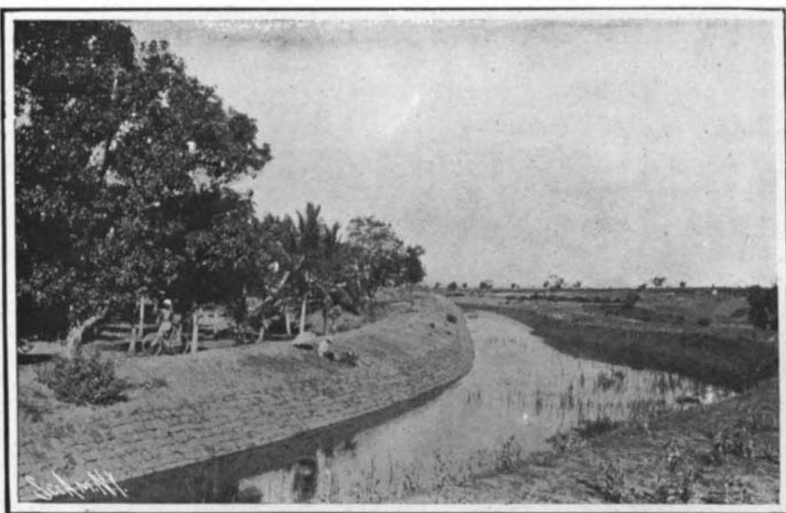
Section of Right Bank, Main Channel 30 Feet Wide at Water Level by 20 Feet at Bottom, Carrying Six Feet of Water.
