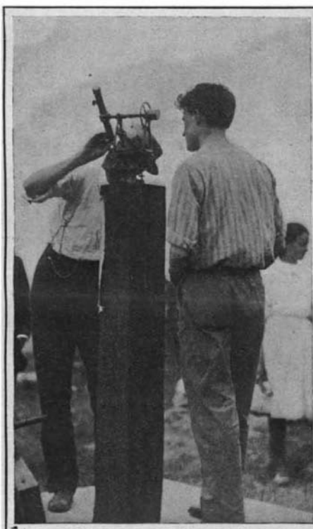
Measuring the Altitude with the Theodolite.
