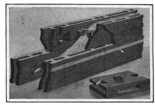
BUILDING BLOCK FOR CONCRETE CONSTRUCTION.
