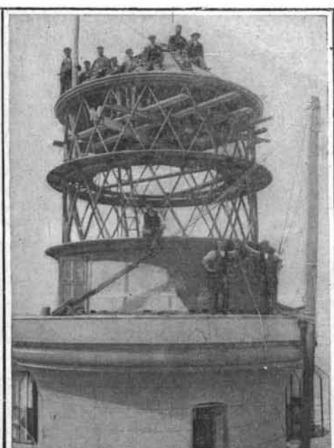
The Lantern in Course of Construction.
