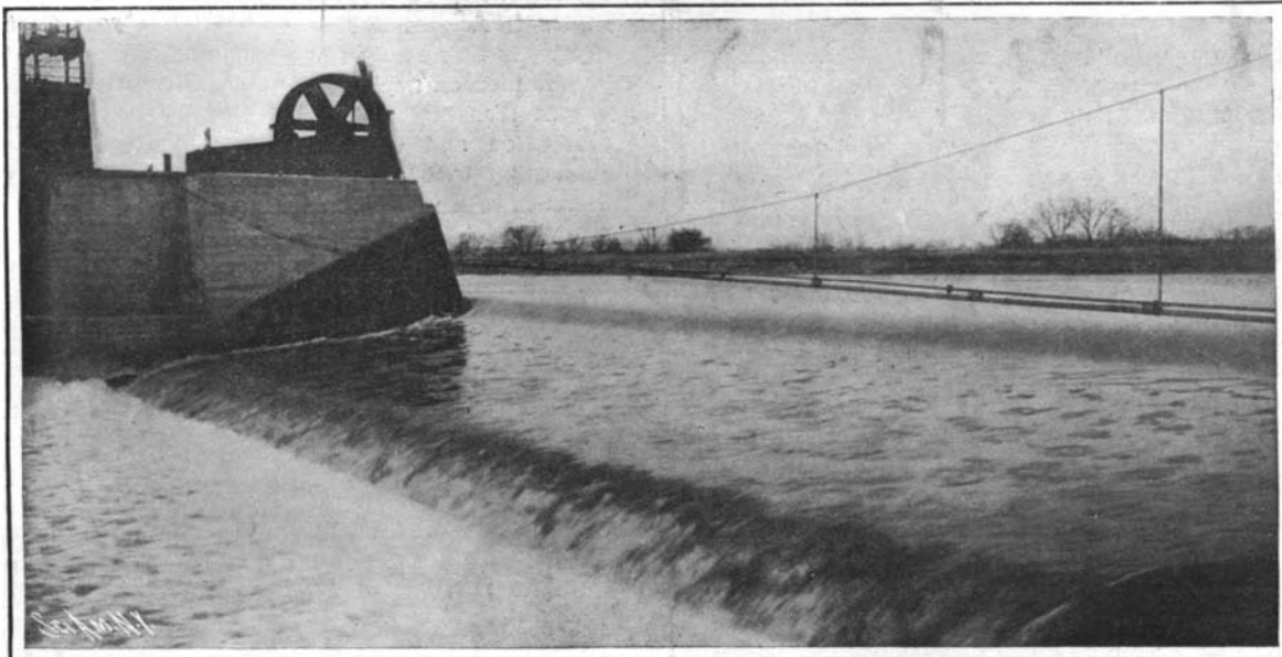
The Bear Trap Dam of the Chicago Drainage Canal.
