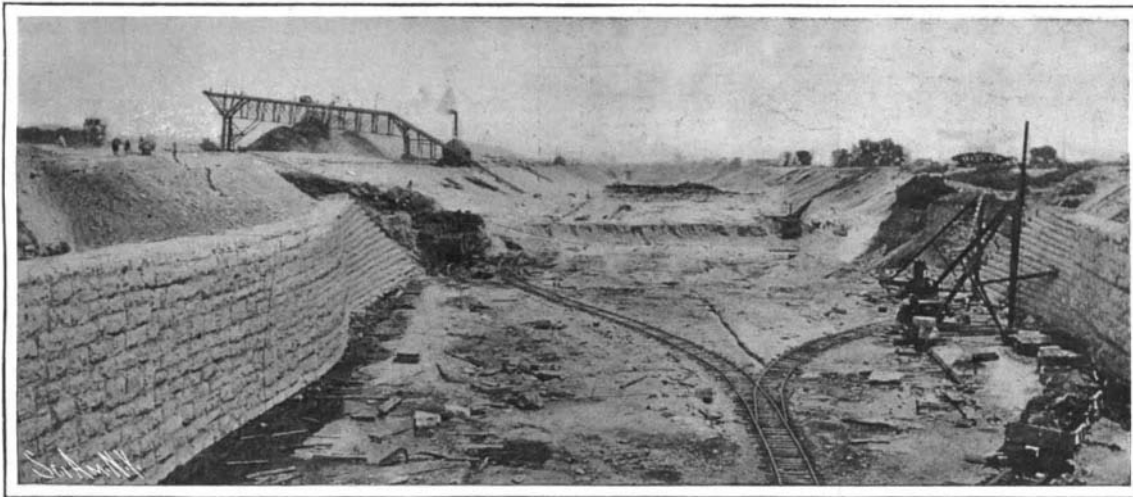
Work on Earth and Rock Sections at Willow Springs.
