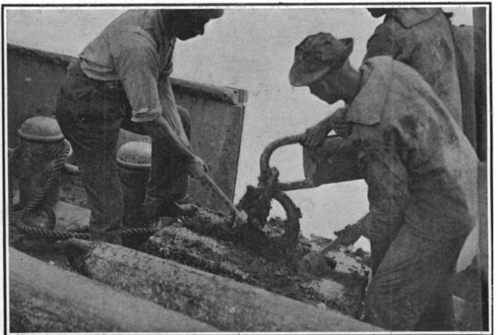
Removing the Spar from Its Anchor.
