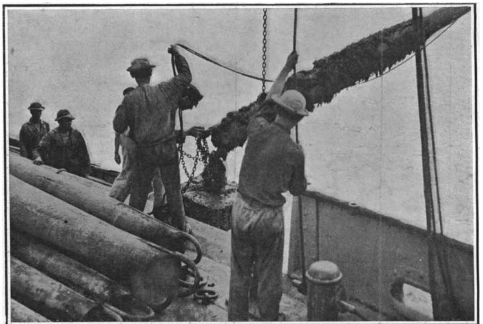
Hoisting a Spar Buoy Aboard the Tender.
