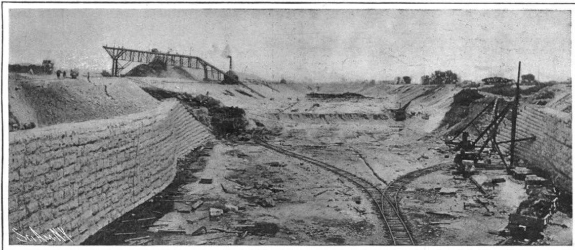
Work on Earth and Rock Sections at Willow Springs.
