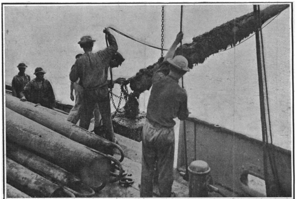
Hoisting a Spar Buoy Aboard the Tender.
