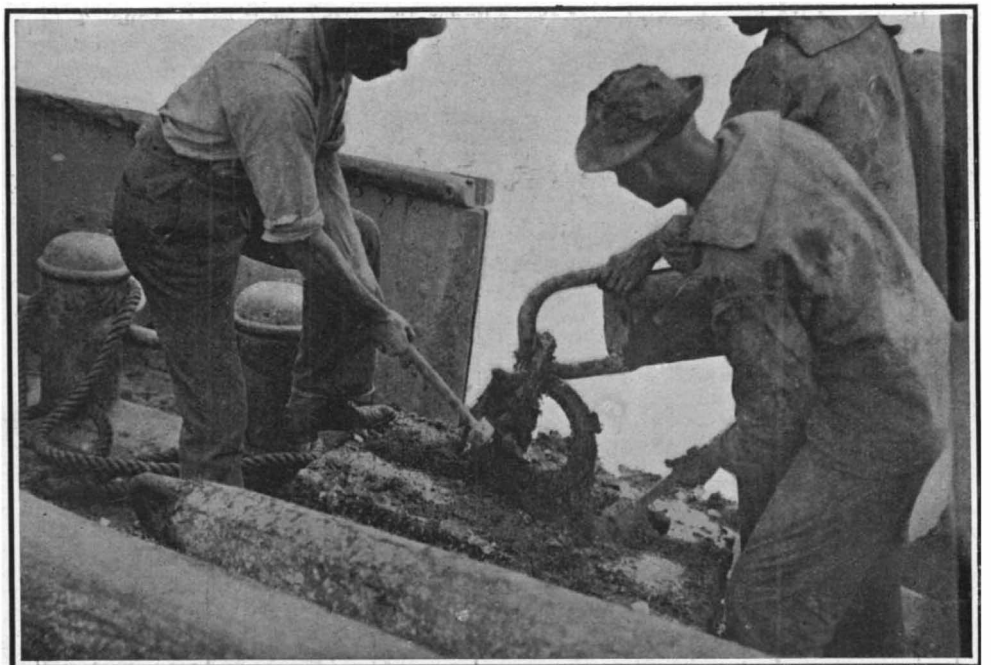
Removing the Spar from Its Anchor.
