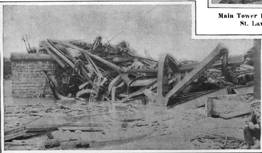
Wreck of Anchor Span, Viewed from the West. Note Complete Crumpling Up of Compression Members.
