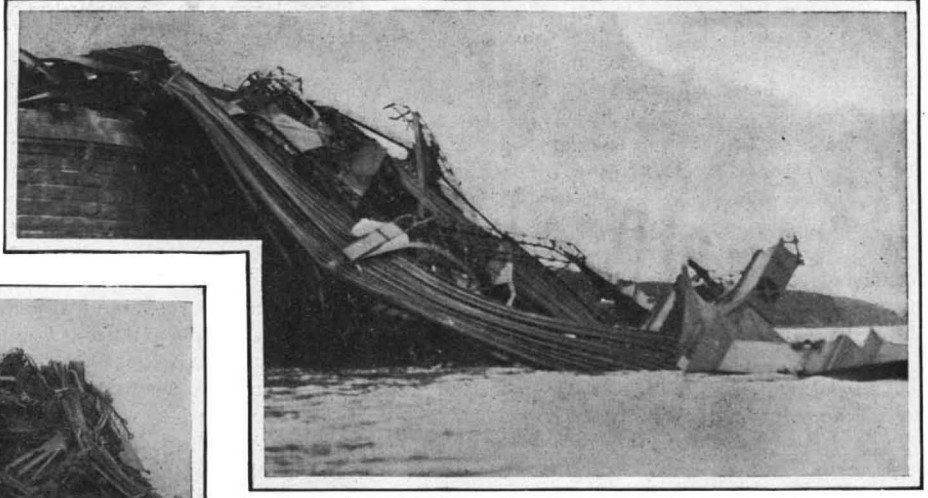
The Top of 315-Foot Main Tower With Top-Chord Eye-bars Still Attached; Viewed from the River.
