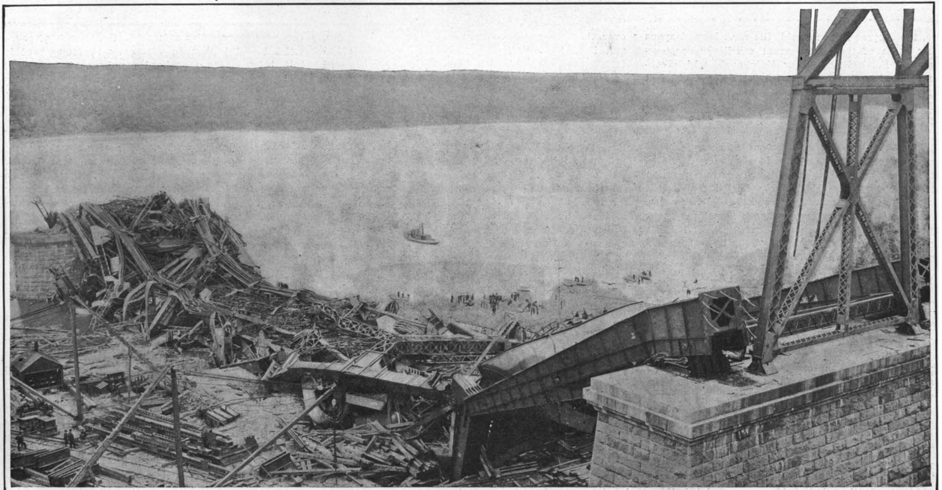
Note the two lines of the top-chord eye-bars, still pinned together, and stretching continuously across the mass of wreckage. General View of the Wreck, Showing How the Trusses Fell in Their Own Vertical Planes. FALL OF THE QUEBEC BRIDGE—THE GREATEST BRIDGE DISASTER IN HISTORY.—[See next page.]
