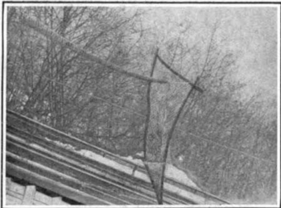
Spring Frame or Buffer for Stopping the Car at the End of Its Course.
