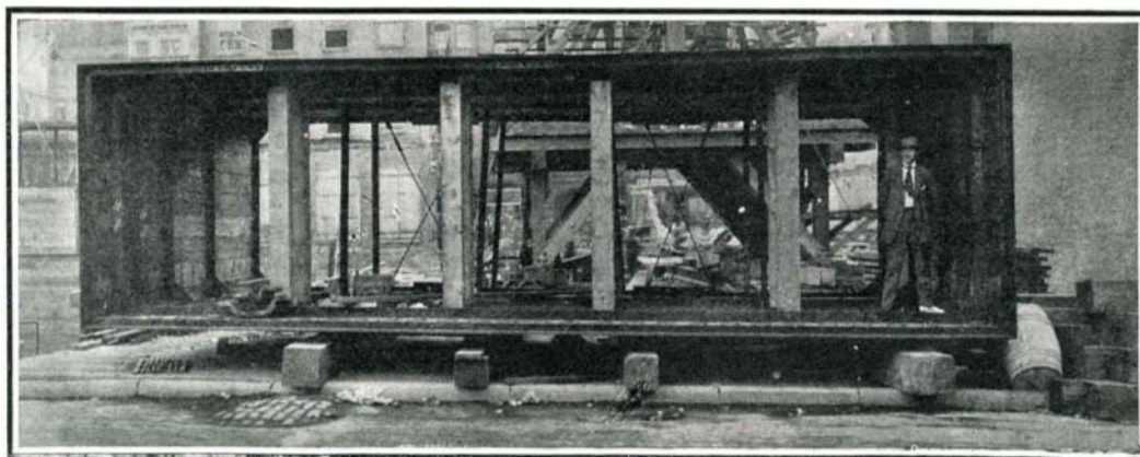
One of the Caisson Forms Used in Building and Sinking the Huge Concrete Wall, 8 Feet Thick and 75 Feet Deep, Inclosing the Foundations of the Cortlandt Street Terminal Station.
