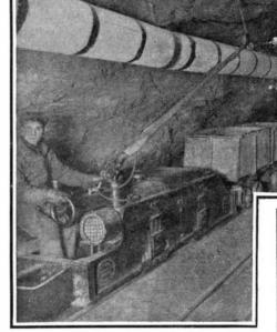
Electric Locomotive Hauling Excavated Material in Hudson Companies' Tunnel Station, 85 Feet Below Present Pennsylvania Railroad Station,
