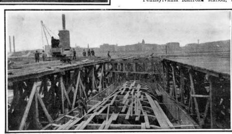
Cut and Cover Work on the Section of Tunnel Connecting the Jersey City Terminal Stations.
