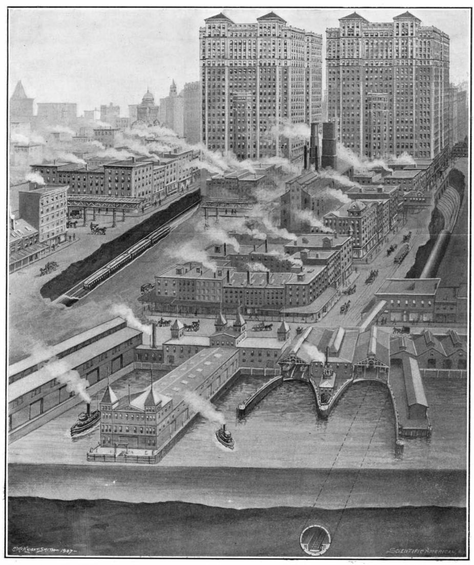
The trains from Jersey City will enter Manhattan by the tube shown in the foreground. The single track will diverge into five tracks, which will swing to the left and enter a six-platform station below the large building shown in the background. This building, 22 stories high, will be nearly three times larger than any existing office building and will house 20,000 people. Trains return to Jersey City by the tunnel shown at the left of building,
