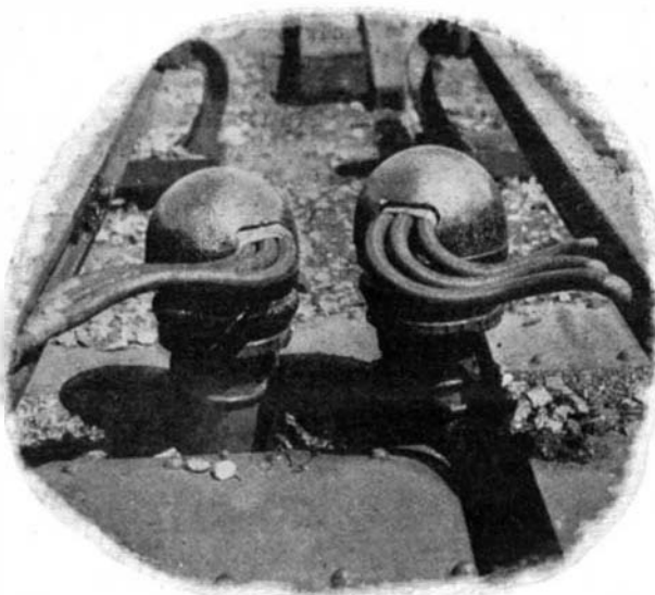
Third-Rail Jumper Connections Used at Cross-Overs.
