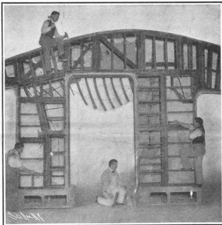
The Skeleton is Mounted in Sections Which Can be Taken Apart and Reassembled.
