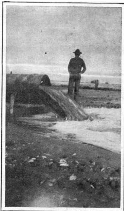
The Discharge End of the Pipe.
