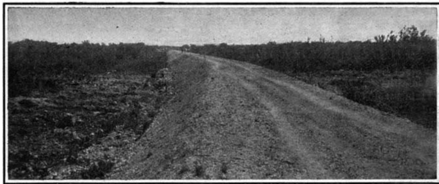
A ROCK FILL ALONG THE ROAD AT KEY LARGO. MORE THAN FIFTY MILES OF SUCH EMBANKMENTS MUST BE BUILT.
