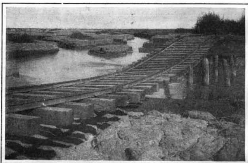
Railroad Tracks Undercut by the Colorado.
