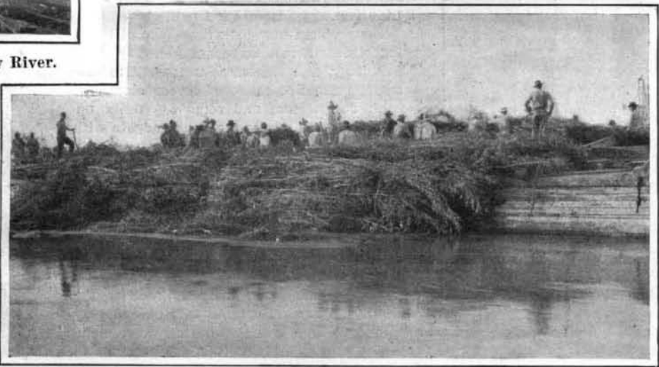
Making Brush Mats for Closure Works.
