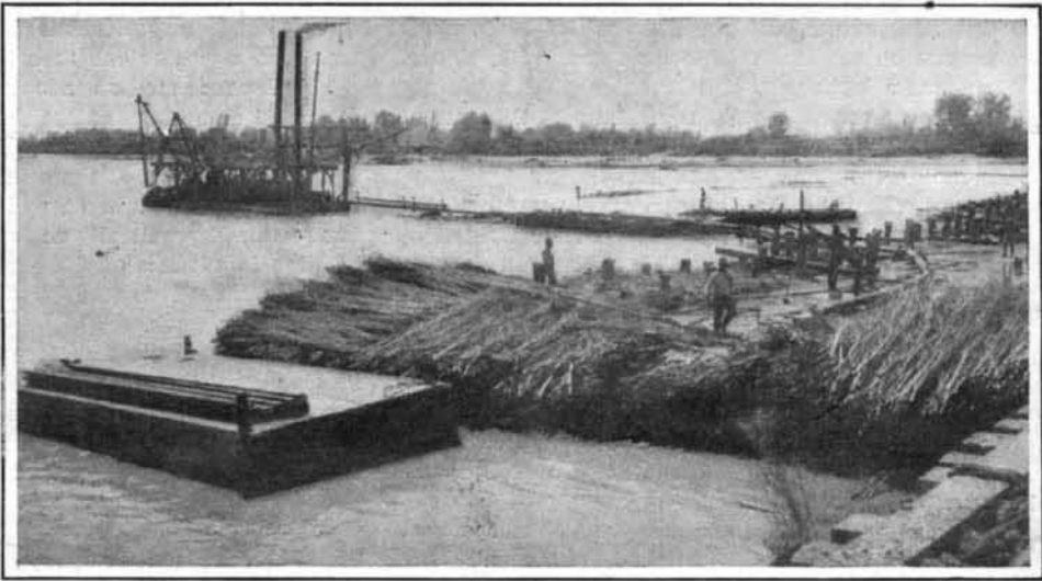
Constructing Mats for Closing the Break.
