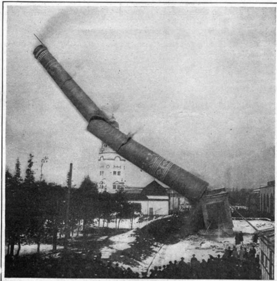
Fig. 3.—As It Fell the Stack Slid From Its Pedestal and Broke Into Several Parts.
