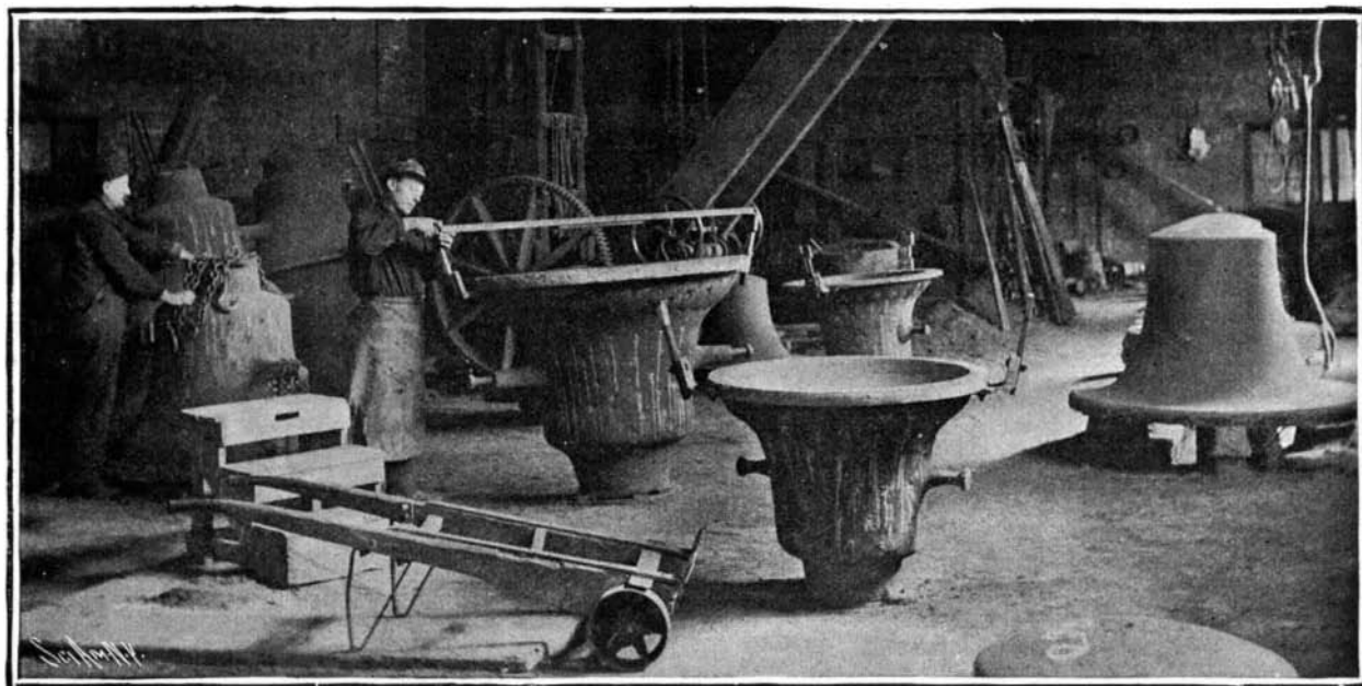
Fig. 3.—The Foundry, Showing Flasks and Cores.
