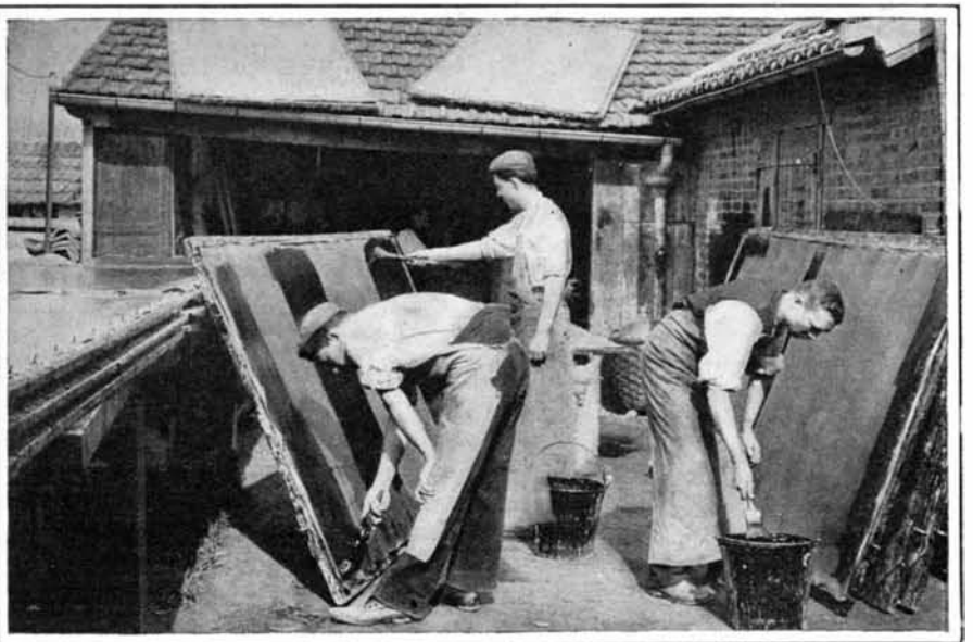
Coating Muslin with Shellac for Foundation.
