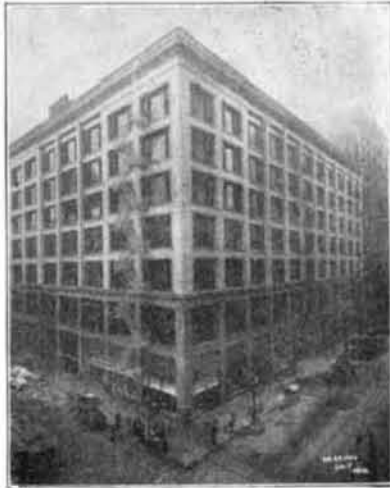
One of Chicago's most famous Department Stores—Fire-proofed throughout by the National Fire Proofing Company.
