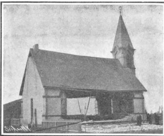
The Walls Blown Out.
