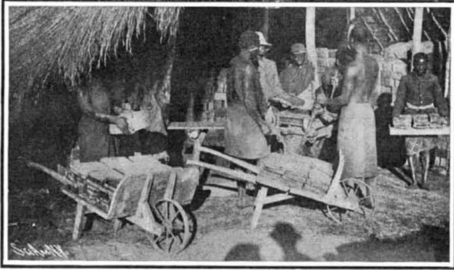
An Immense Shed of Thatched Grass Protected the Bricks.
