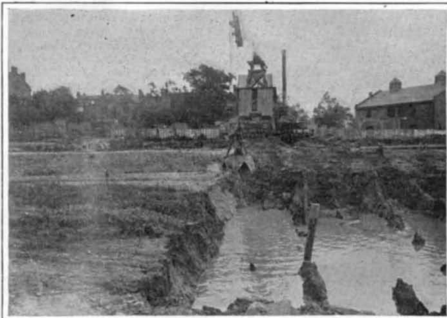
Breaking Ground. An Orange Peel Shovel Beginning the Work of Excavation.
