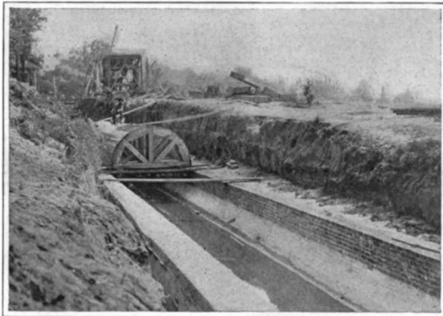
The Dry Land Continuation of the Outfall Sewer.
