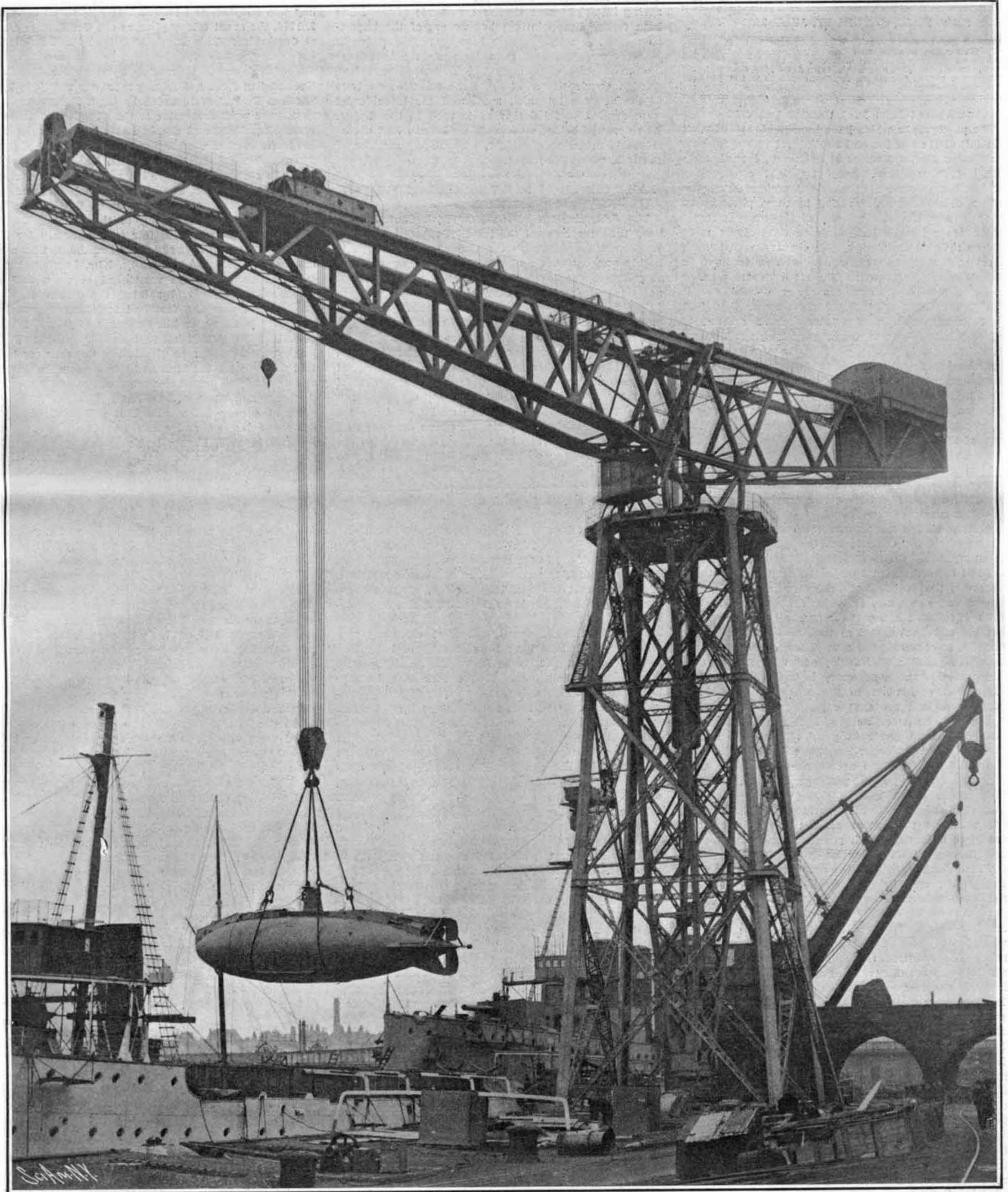
LIFTING A BRITISH SUBMARINE BOAT WITH A 150-TON ELECTRIC CRANE.—[See page 67.]
