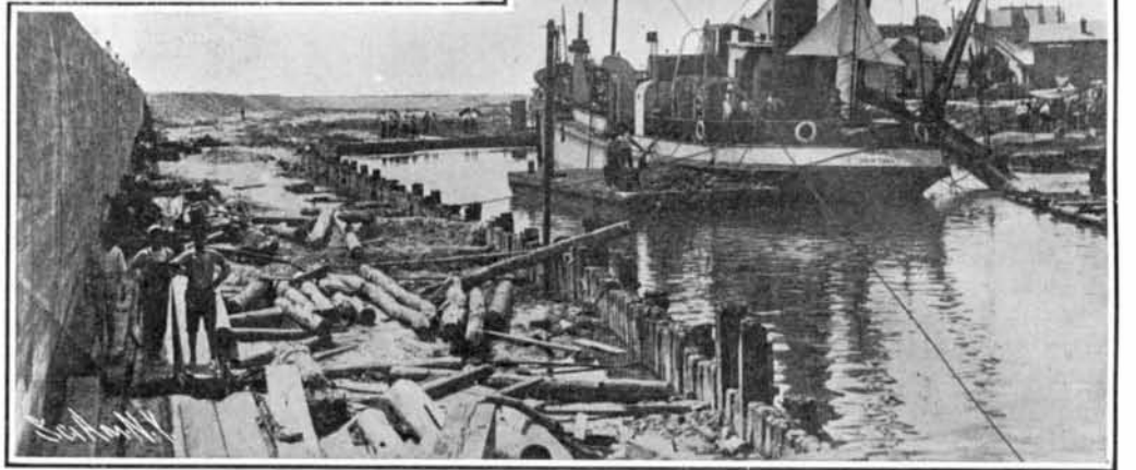
The "Holm" Commencing to Dig the Distributing Canal. The Sea Wall is on the Left. The Canal Pierces the Heart of the Town. The Dredgers Steam up It and Discharge Their Loads under the Houses.
