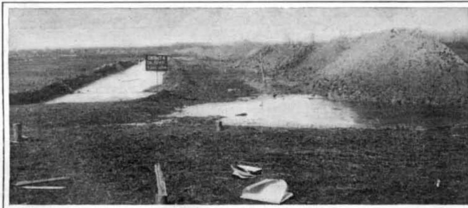
Embankment Thrown Up by Mechanical Excavator.
