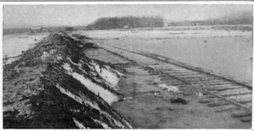
Excavation Partly Completed on Eastern Division.
