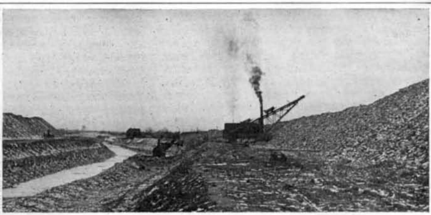
General View of Excavation, Showing Deep Cut Near Rochester.
