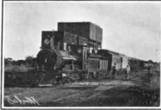
Temporary Wooden Water Tanks and New Overhead Cast-Iron Tank of 30,000 Gallons Capacity.
