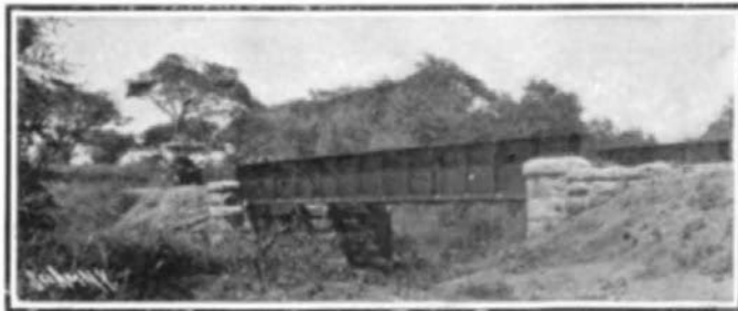
Type of Bridge Adopted for 50-Foot Spans on the Victoria Falls Section.
