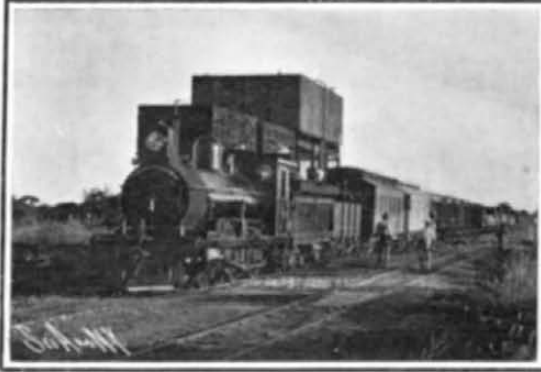
Temporary Wooden Water Tanks and New Overhead Cast-Iron Tank of 30,000 Gallons Capacity.
