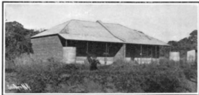
Typical Double Gangers' Cottage.
