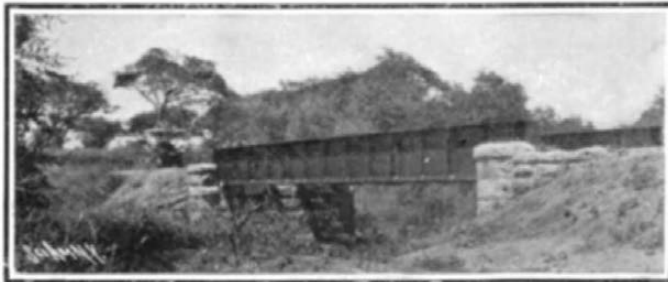
Type of Bridge Adopted for 50-Foot Spans on the Victoria Falls Section.
