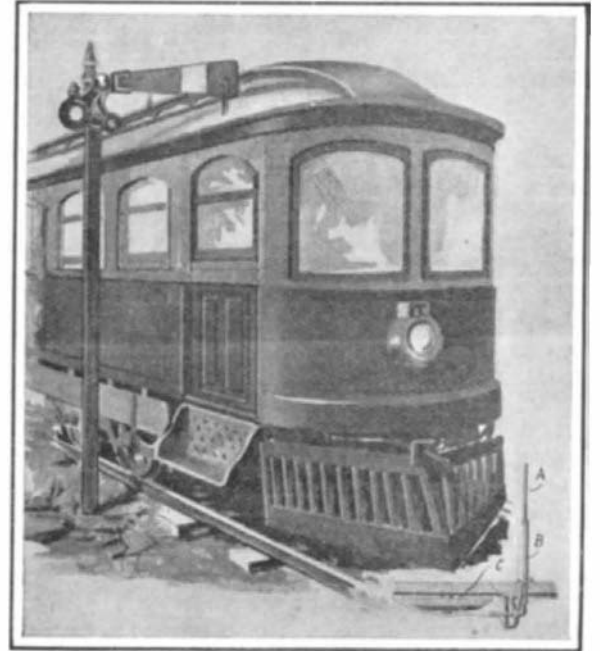
RAILWAY SIGNAL DEVICE.
