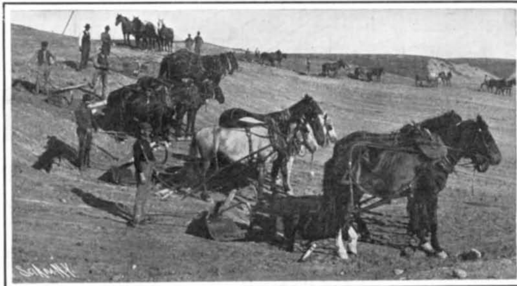
Team Excavations on the Main Canal.
