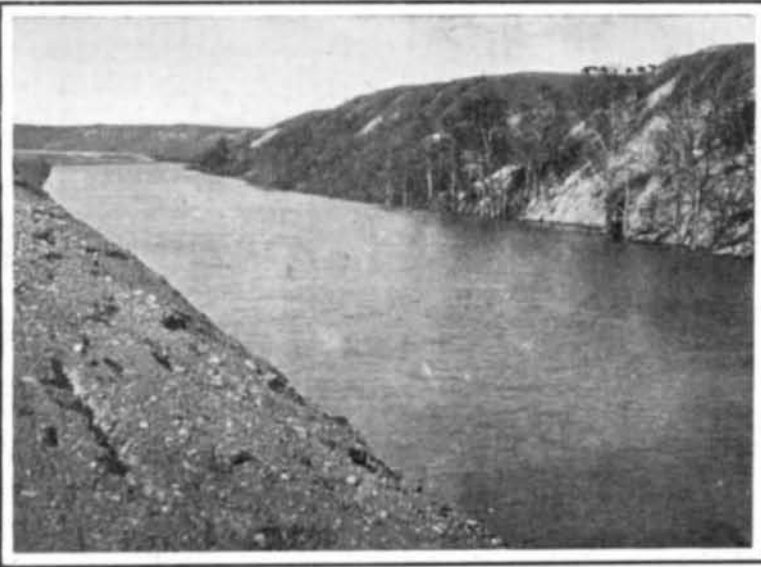
Along the Main Canal.
