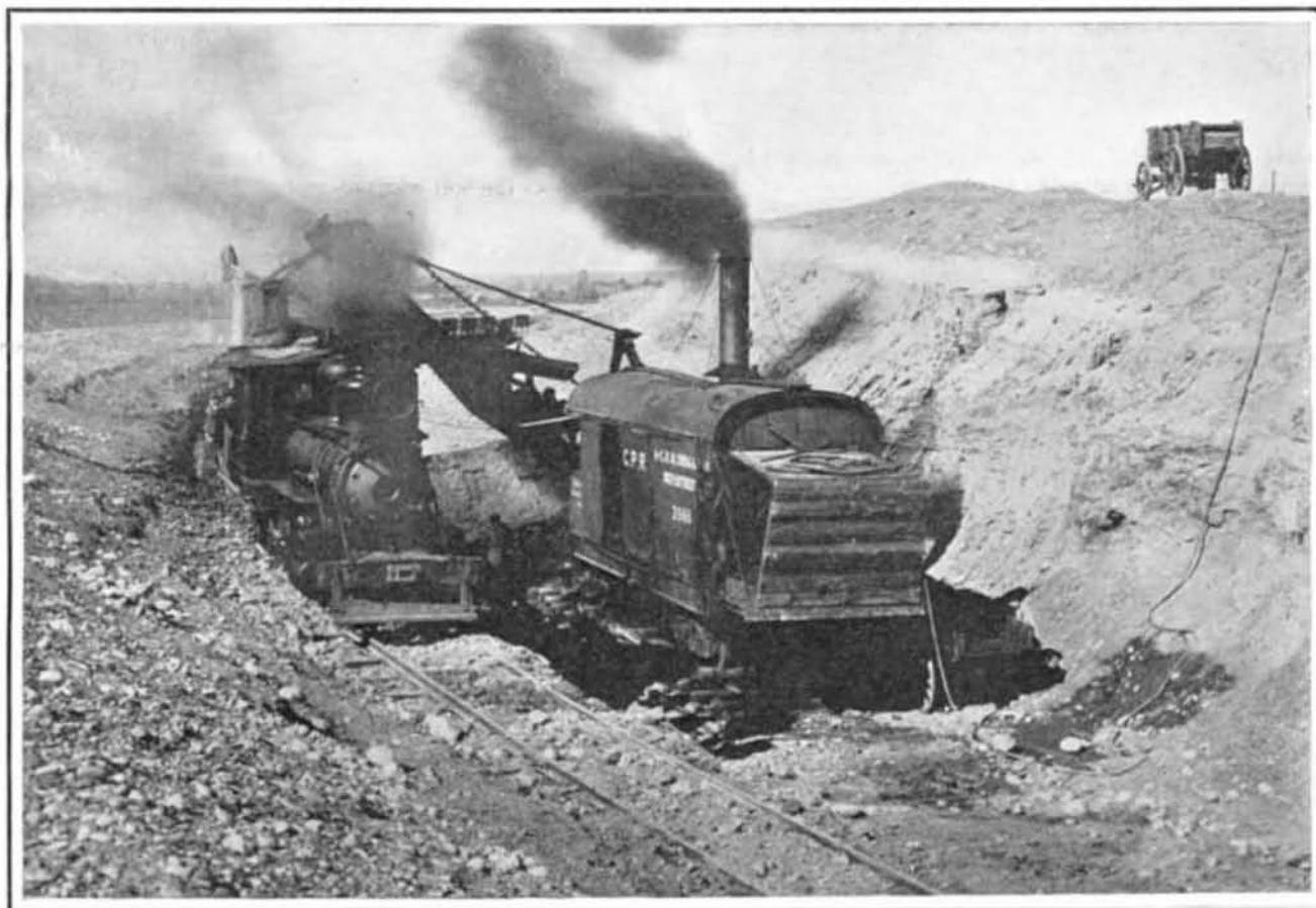
A Steam Excavator at Work.
