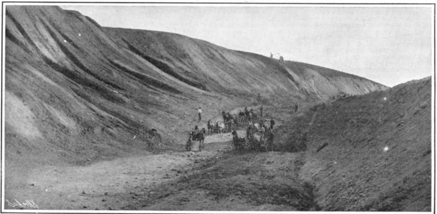
A Huge Cut on the Main Canal.
