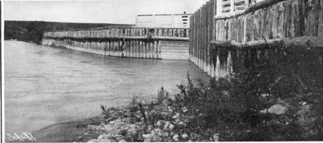
Headgate and Piles for Protecting the Banks of the River.
