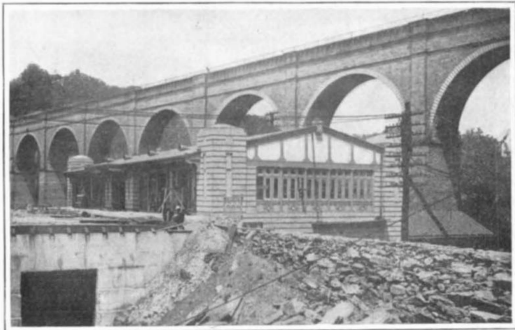
The tracks are built within the concrete structure, and the station is placed transversely above it. The sloping approach in the foreground is the unfinished street, which is to be carried over the tracks.
