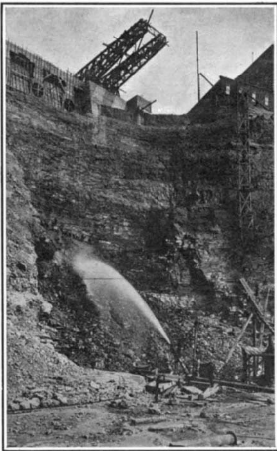
Excavating the Power House Site.
