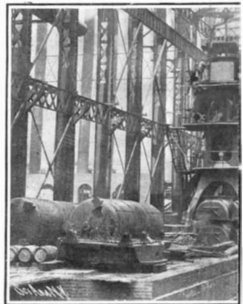
Erecting One of the Blowing Engine Furna
